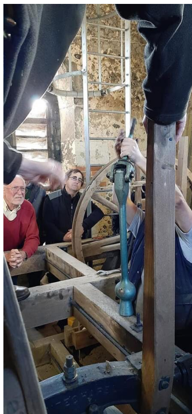
Work in the tower
